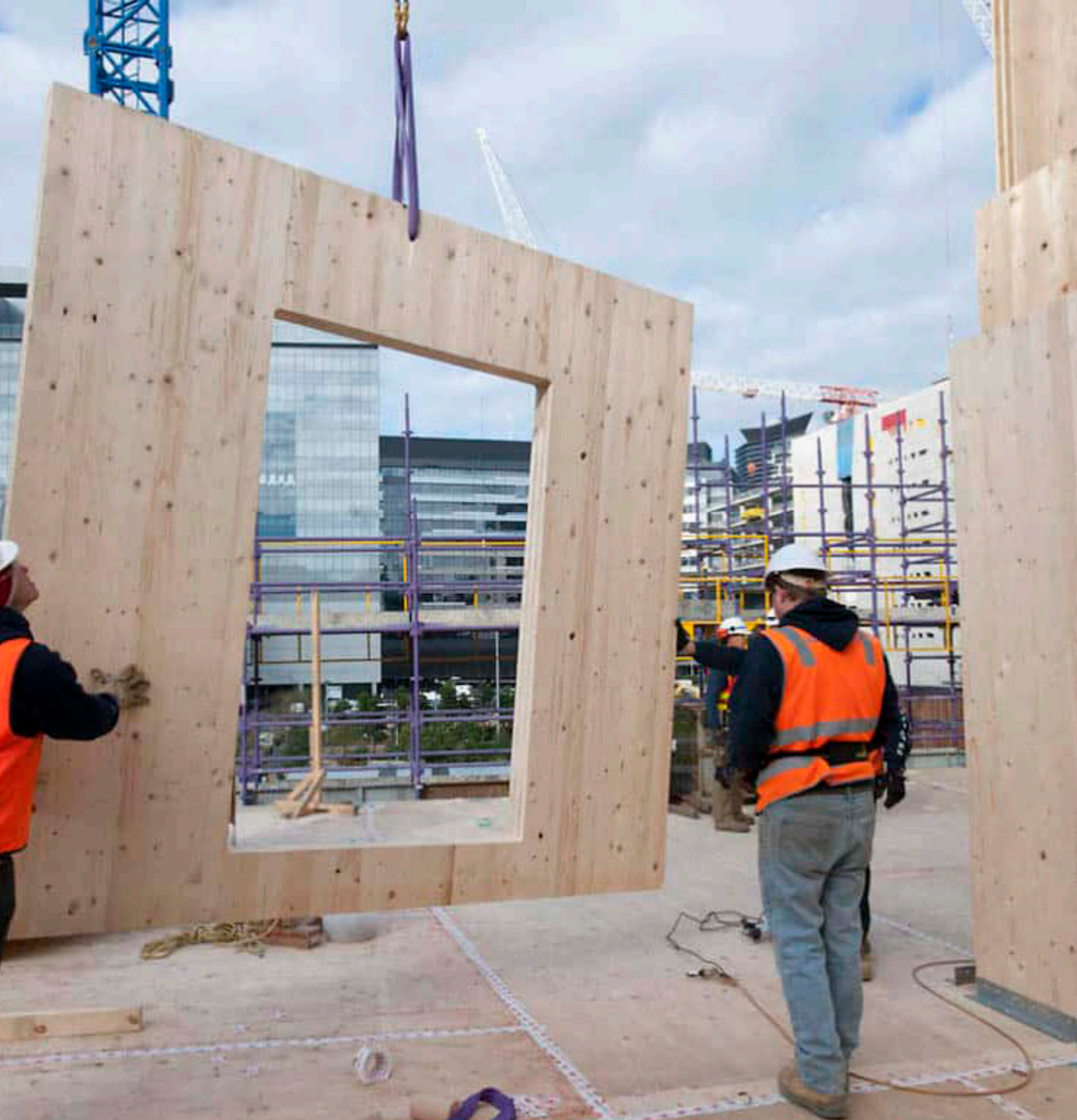
https://buildingconnection.com.au/wp-content/uploads/sites/5/2016/07/Forte-CLT-panel-installation.jpg Peter Williamson
